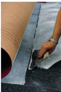
The next step is to press once more the wall edges with a roller, to trim them and then press them again against the adhesive. Then the whole surface has to be rolled and the seams have to be cut. After approximately 30 minutes, the seams and edges have to be pressed again.
