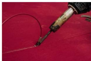
The processing temperature is around 400 - 450 °C. Choose a suitable working speed so that ideally the welding rod is running into the milled groove. This corresponds to a running speed of 2.5 - 3.0 m/mm.
