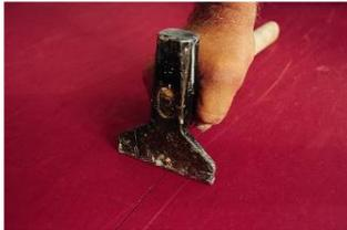
Depending on the climatic conditions, half an hour after laying all the seams and edges have to be pressed down thoroughly once more with a heavy hammer.
