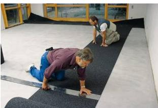
The laying direction of the elastic mat should be the same as that of the top covering. It is recommended that the linoleum be laid out from the central axis of the room towards both walls. Head seams, if required, must be offset by 50 cm. Lengths running towards the face wall should be measured and laid out at the end.
