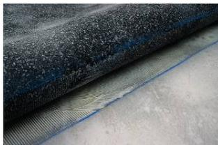
Then lay the mat lengths by smoothing or rolling them into the wet adhesive within the period specified by the manufacturer. The amount of time required to lay depends on the ambient temperature, the air humidity, as well as the absorbency and moisture of the subbase. Avoid trapping air when laying the mat. If air bubbles occur, press them out sideways.
