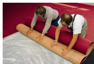
The edges at the ends of each length (at the wall) have to be pressed and rolled against the adhesive bed.
