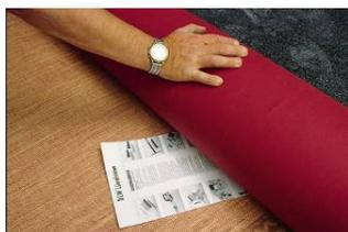
After determining the ambient temperature, sub floor temperature and air humidity, any dirt in the area must be removed using a vacuum cleaner. The linoleum can then be rolled out.
