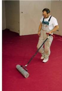
It is recommended that the surface be inspected with a hammer after rolling to hear whether there is air trapped. If there is it must be let out through a small incision in the linoleum. If in doubt, place weights on these areas.
