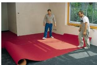
Measure the exact dimensions of the room, and determine the middle of the area by spanning string across both its width and its length.
